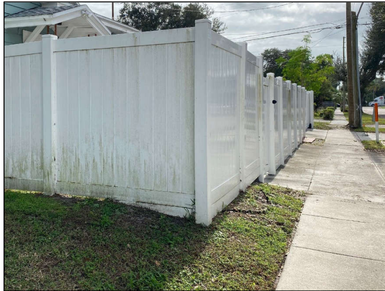
Figure 9: Deteriorated and stained vinyl within subject district.
