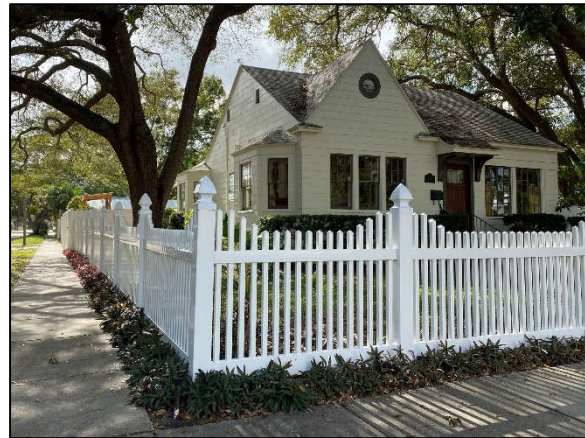
Figure 6: Lower (3-to 4-foot) vinyl fencing with decorative design and higher transparency at front and street side yard of property in subject district
